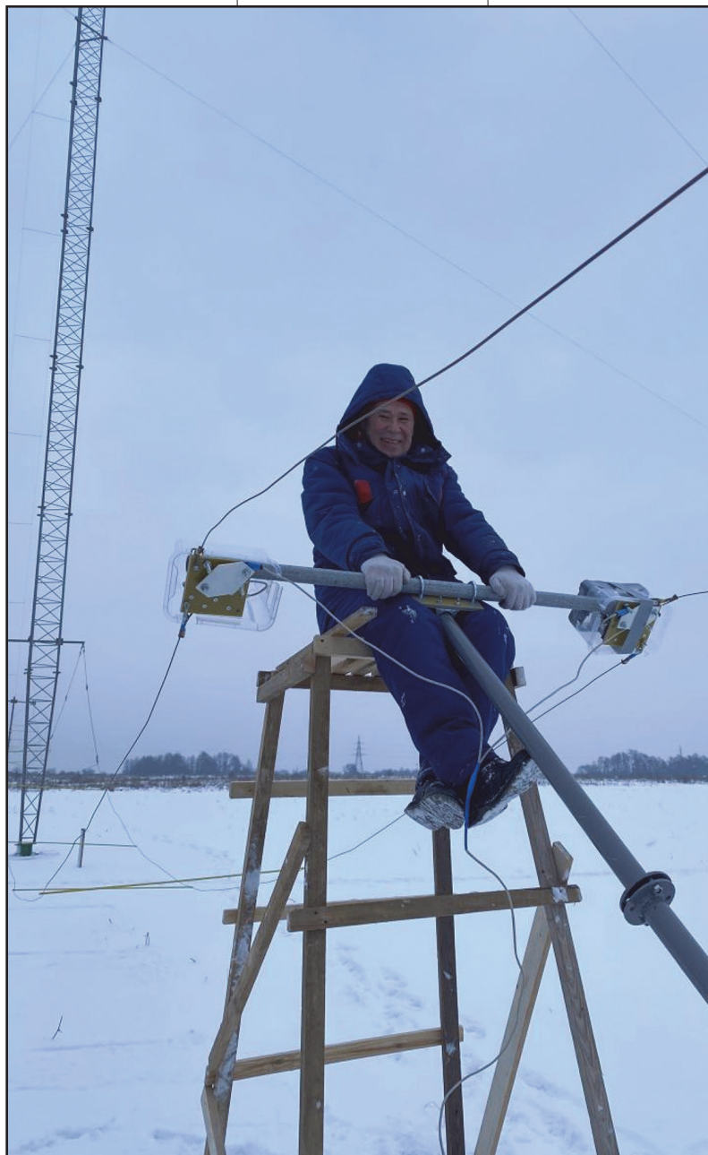
Radik, RT2F, is either riding a dog sled, or installing the UA2FW director switch.
